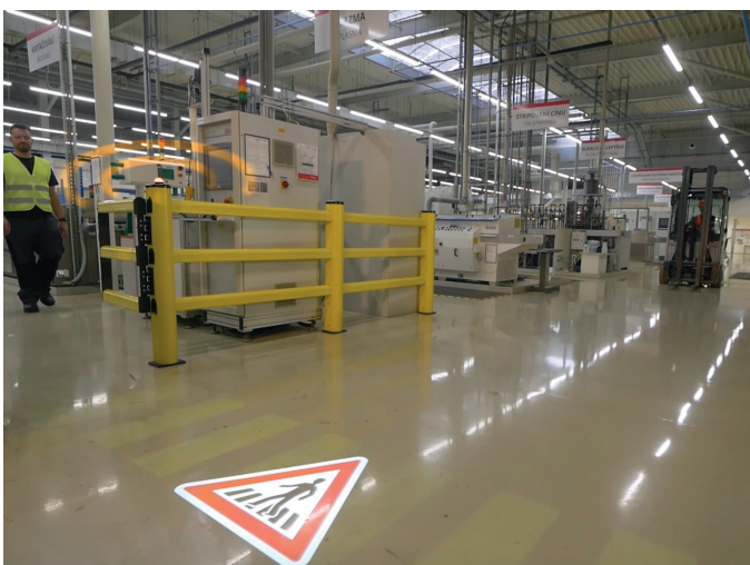
warning zone - connectivity to LED floor marking (symbol changing)
