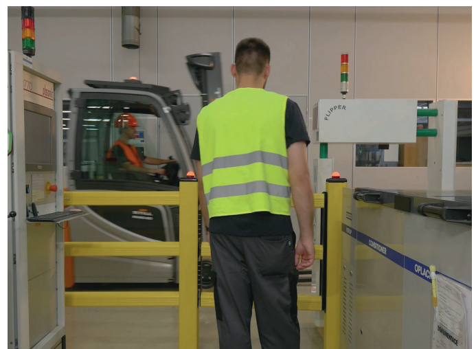
danger zone - magnetic lock
