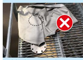
A hole with its cover removed is not visible beneath this cloth. A potential safety hazard.
